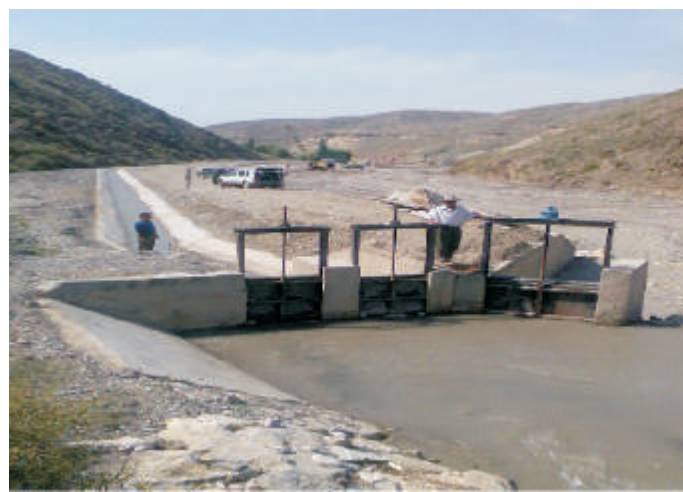
“Besh-Baatyr” WUA. Head intake structure at Zhin-Zhigen canal. before and after rehabilitation
