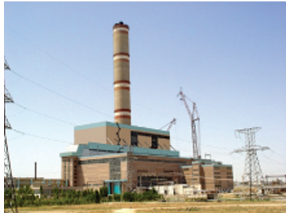
The Talimarjan Power Project. ADB supported the Talimarjan Power Project that added 900 MW-capacity steam-gas turbines (photo by Talimarjan Project Team).
